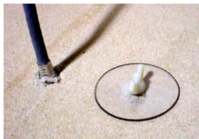
View of Antenna Above Ceiling Tile
